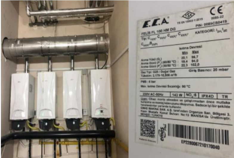
Figure 7. The general view of the wall-mounted condensing boilers of the ISP building heating system.
