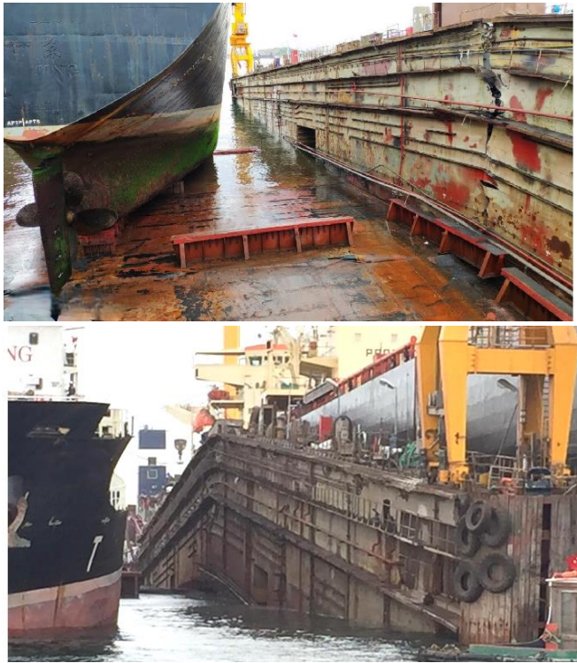
Figure 2. A floating dock broken at the midsection (URL1, URL2).
