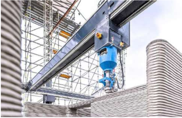
Figure 1. 3D cementitious material printing (PERI, 2020).
