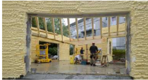
Figure 4. Batiprint3D House where polyurethane foam is used as a mold in 3D printing (Nadarajah, 2018)
