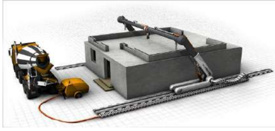
Figure 2. Contour Crafting 3D printing (Anonymous, 2022a).
