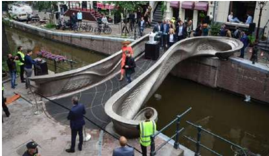
Figure 6. 3D-printed stainless steel footbridge/Amsterdam (MX3D, 2021).
