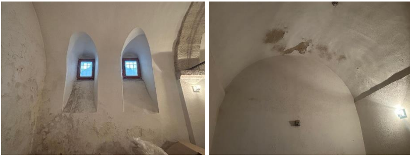
Figure 15. Deteriorations observed in the building after the restoration process (Sezer,2024)
