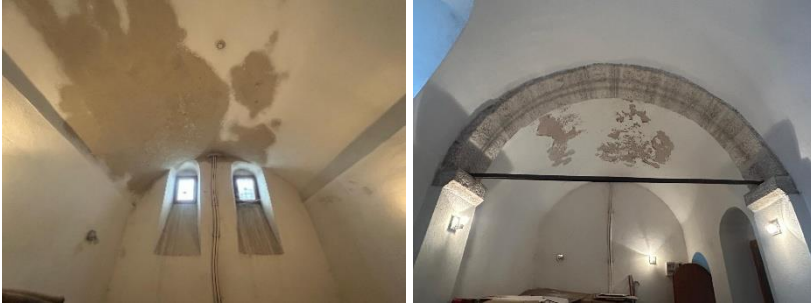
Figure 14. Deteriorations observed in the building after the restoration process (Sezer,2024)
