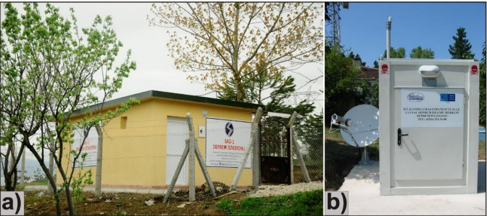
Figure 3. Different types of built seismic stations a) reinforced concrete structure (SAÜ Emarc, 2023) b) Cabin (KOERI, 2023)
