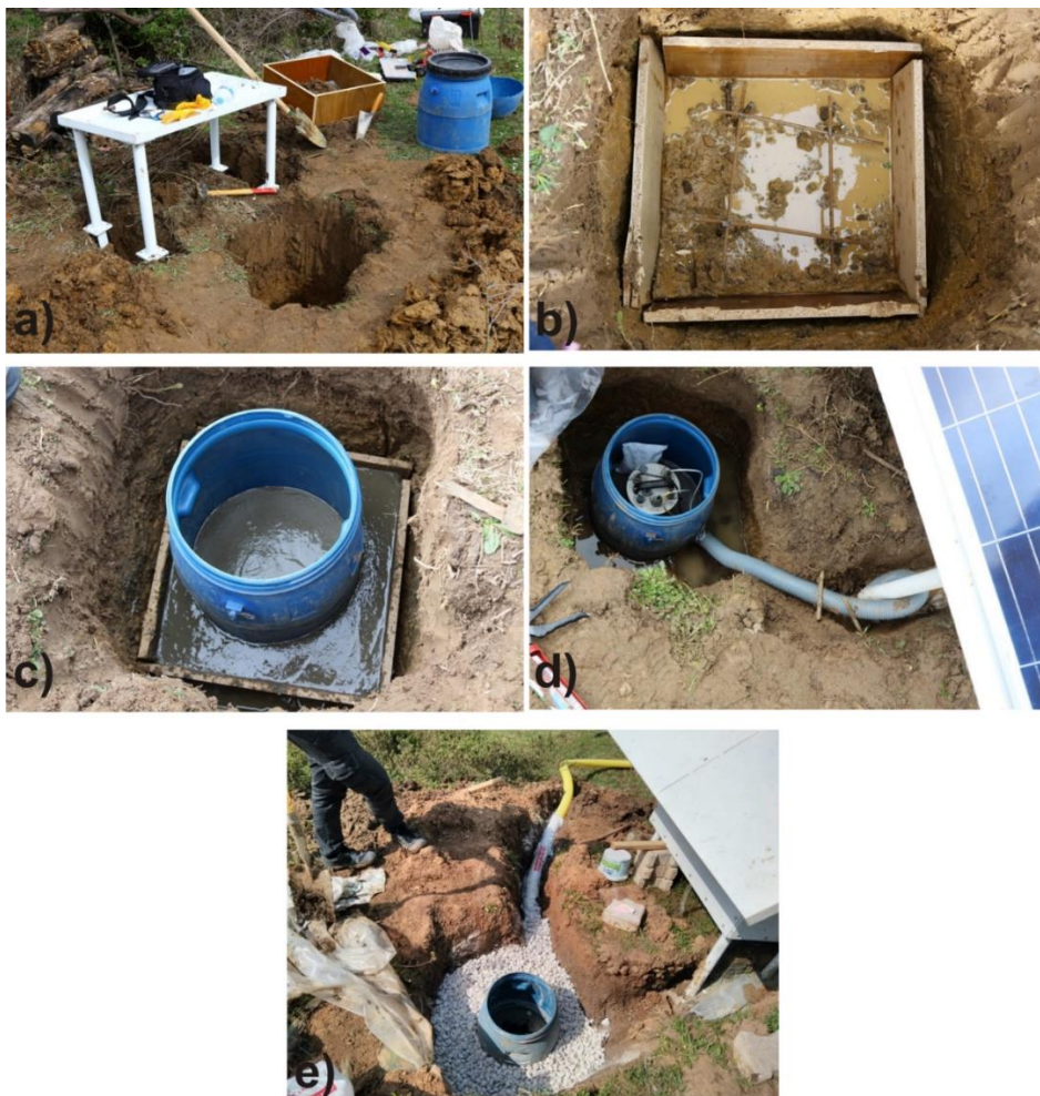
Figure 7. Stages of station setup a) The holes dug for the installation of the station b) The mold and iron prepared for the concrete table where the sensor will be placed c) The construction phase of the environment in which the earthquake sensor will be placed d) The connections prepared for the installation of the earthquake sensor e) Drainage process
