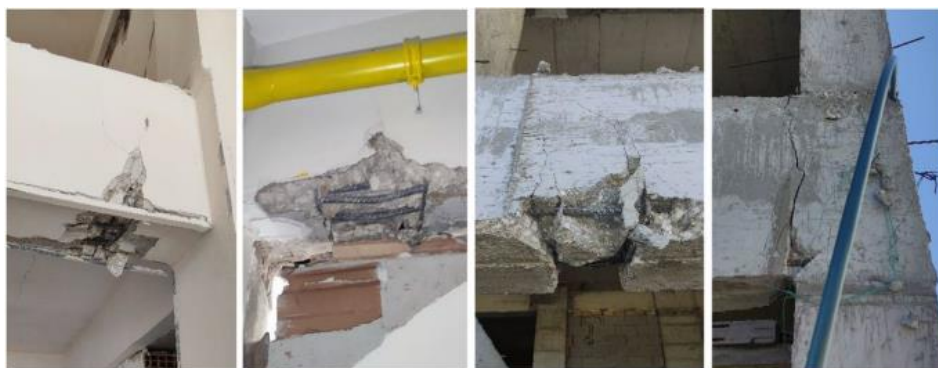
Figure 6. Flexural crack in a beam [50]
