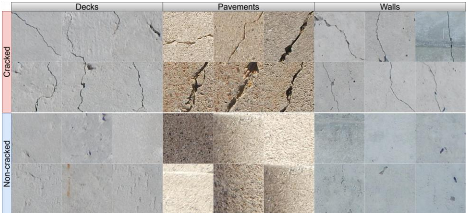
Figure 1. Sample images from the dataset for cracked and non-cracked classes across different concrete structure types (Decks, Pavements, and Walls).
