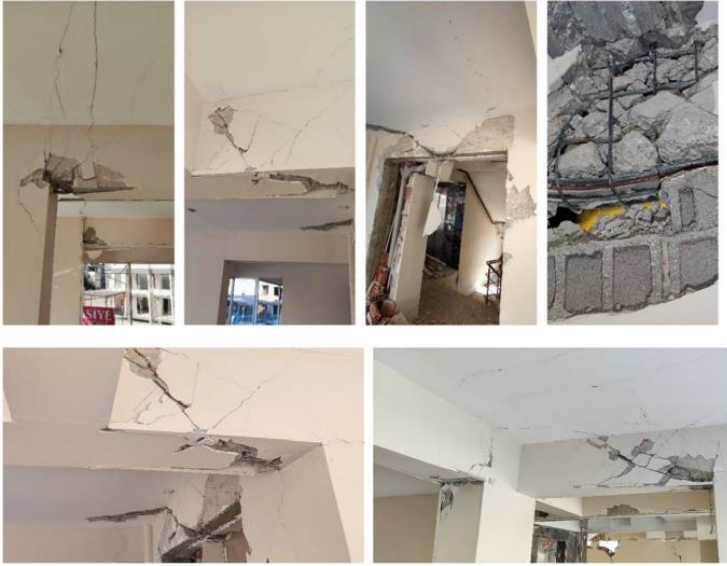
Figure 8. Shear cracks in beams [50]
