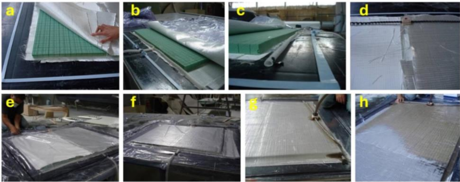
Figure 8. VARIM production stages of sandwich composite material (GCG Yacht Manufacturing Industry Inc., Sarnıç, İzmir), a) Placement of glass Fiber and foam materials into the mold b) pulling of spiral hoses, c, d) Installation of resin and vacuum hoses, e) Placement of vacuum nylon, f) Applying sealing paste, g, h) Opening of resin feeding line and resin impregnation.
