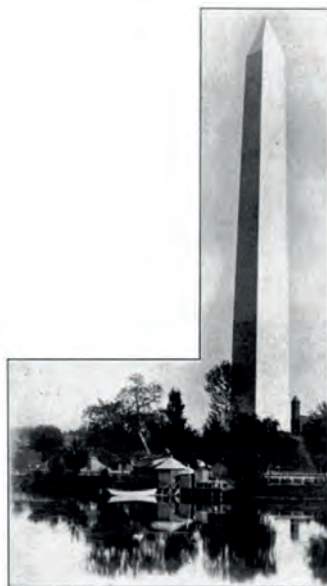
FIG. 239.—WASHINGTON'S MONUMENT. HEIGHT 555 FEET, 5½ INCHES. HIGHEST MASONRY STRUCTURE IN THE WORLD.
