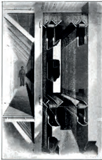
FIG. 264.—EDISON MAGNETIC CONCENTRATOR.
