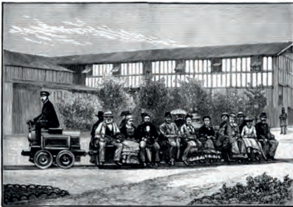
FIG. 33.—SIEMENS' FIRST ELECTRIC RAILWAY.
