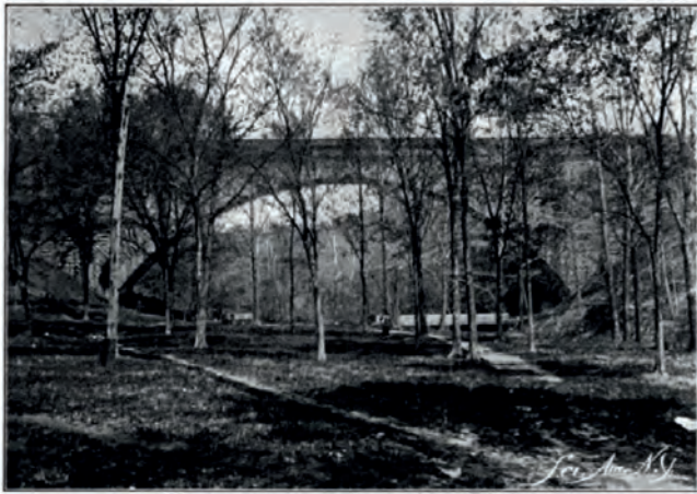
FIG. 230.—CABIN JOHN BRIDGE, NEAR WASHINGTON, D. C. LARGEST MASONRY ARCH IN THE WORLD. LENGTH, 450 FEET; SPAN OF ARCH, 220 FEET; HEIGHT, 100 FEET.
