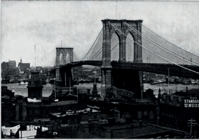
FIG. 229.—THE BROOKLYN BRIDGE. LONGEST SUSPENSION BRIDGE IN THE WORLD. TOTAL LENGTH, 5,989 FEET; SPAN BETWEEN TOWERS, 1,595 FEET 6 INCHES.
