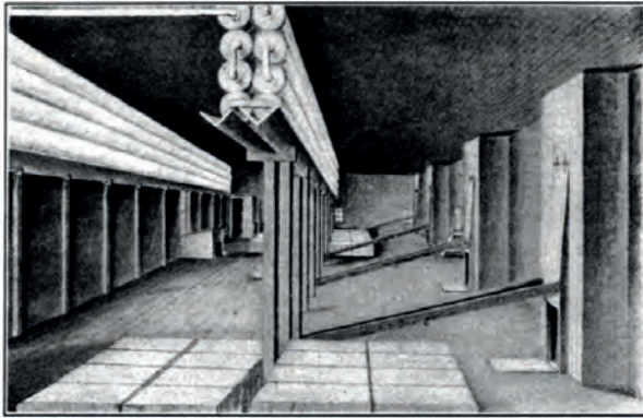
FIG. 298.—STORAGE ROOM OF ICE PLANT.
