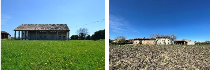
Figure 3: Cascina Rural Houses 6 .
