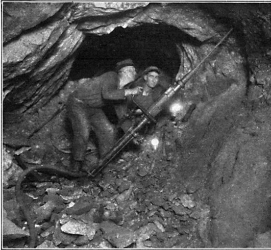
DRILLING WITH COMPRESSED AIR IN A COPPER MINE. The drill also forces a stream of water into the hole to lay the dangerous sulphur-bearing dust. ( Courtesy Sullivan Machinery Co. )
