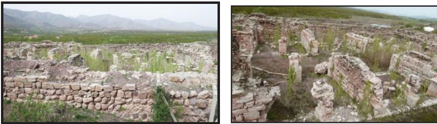
Figure 10: Images showing the current state of the Sevserek Han building (URL3).
