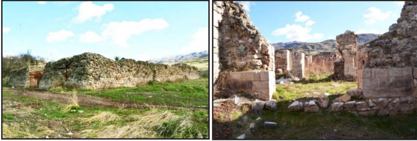
Figure 9: Sevserek Han shows the main wall and its foundations (URL2)
