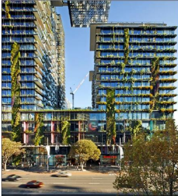
Figure 1. One Central Park (Sydney) vertical garden application
