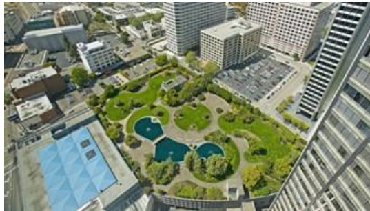
Figure 3: Kaiser Roof Garden (URL 3)
