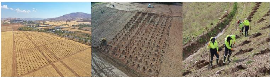
Figure 2. Digging Pits in Afforestation Areas
