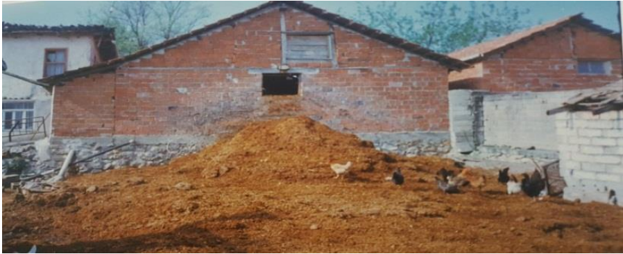
Figure 10. Manure discharge opening in a barn
